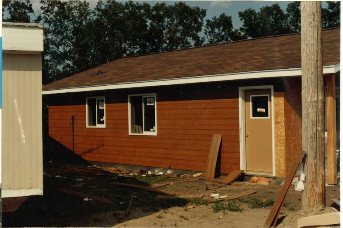
Building of the new campground office and supervisor's house - 1989.
