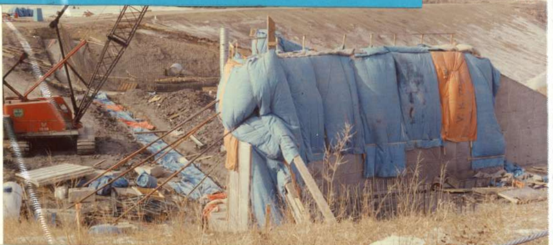
Building of the new spillway and raising of the lake - 1981.
