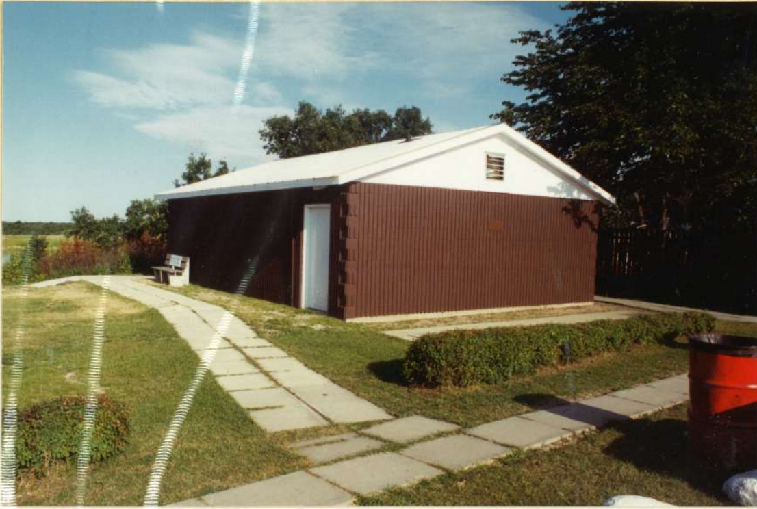
Renovations to camper washroom, 1994.
