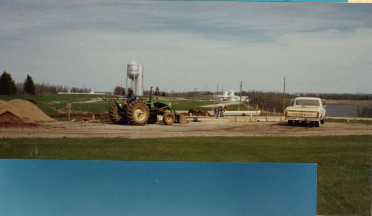
Building the washroom for the new development--1995.
